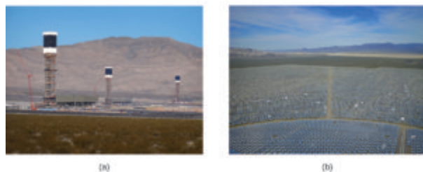
Figure 9 (a) The Ivanpah solar thermal plant uses 170,000 mirrors to concentrate sunlight on water-filled towers. (b) It covers 4000 acres of public land near the Mojave Desert and the California-Nevada border. (credit a: modification of work by Craig Dietrich; credit b: modification of work by “USFWS Pacific Southwest Region”/Flickr)
